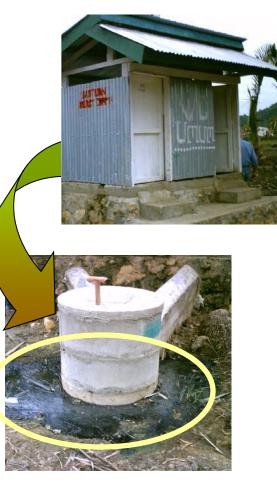
Visual inspection behind the latrine (top) reveals a leaking septic tank (bottom).
